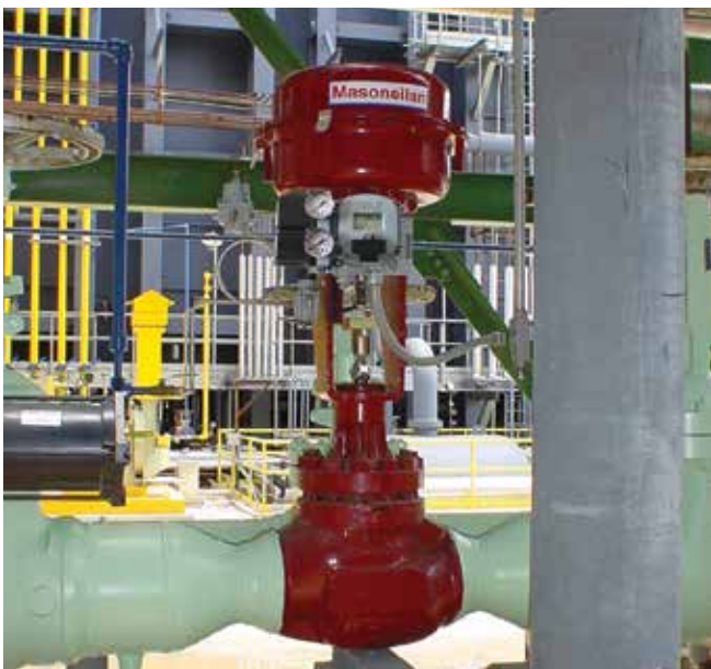
SVI II AP on severe service valve
